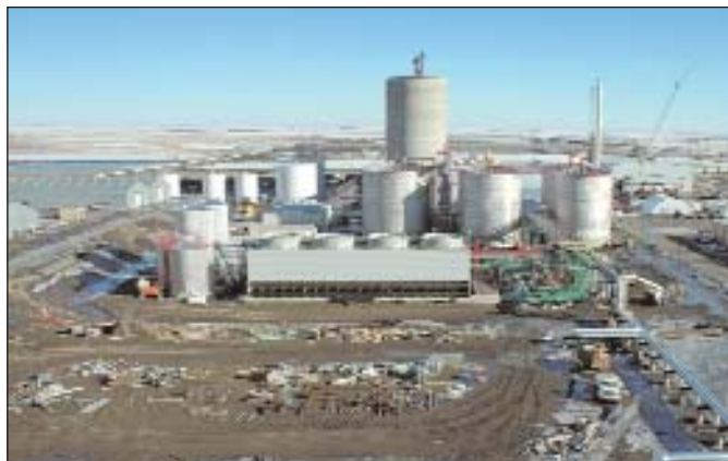
Blue Flint Ethanol, a 50 MMgy ethanol plant that recently started production in Underwood, N.D., is powered by electricity and process steam from the Coal Creek Station power plant.
